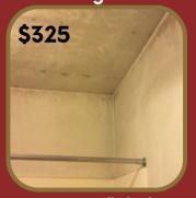
Damage to walls/ceiling from mildew - will require deep cleaning/wall repair
